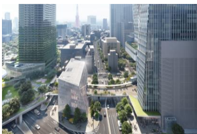
T-Deck above the Sakurada-dori Avenue
