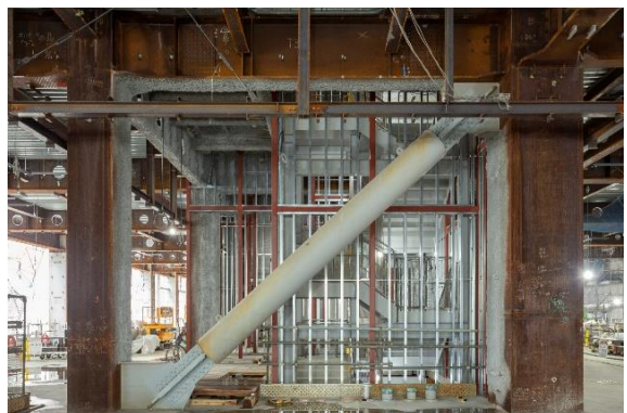
■ Buckling restrained braces
