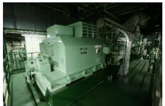
Gas engine generator (rendition)
