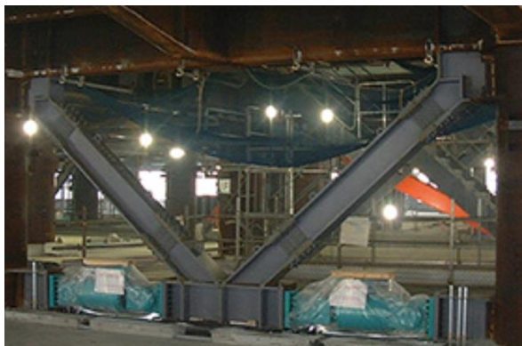
Semi-active oil dampers
