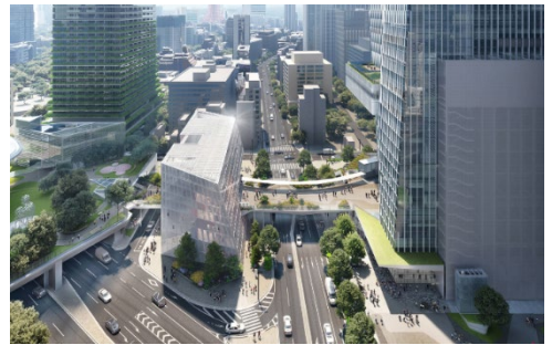
T-Deck spanning Sakurada-dori Avenue
