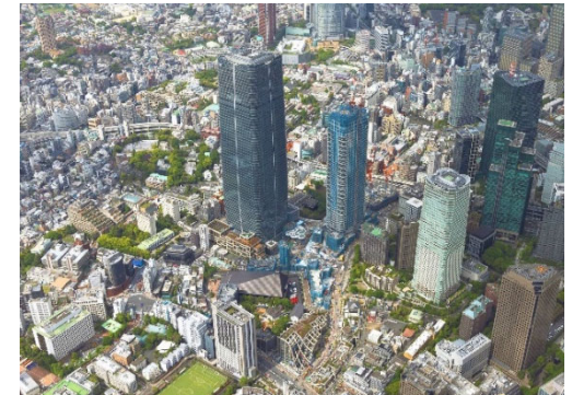
Construction site (April 18, 2023)
