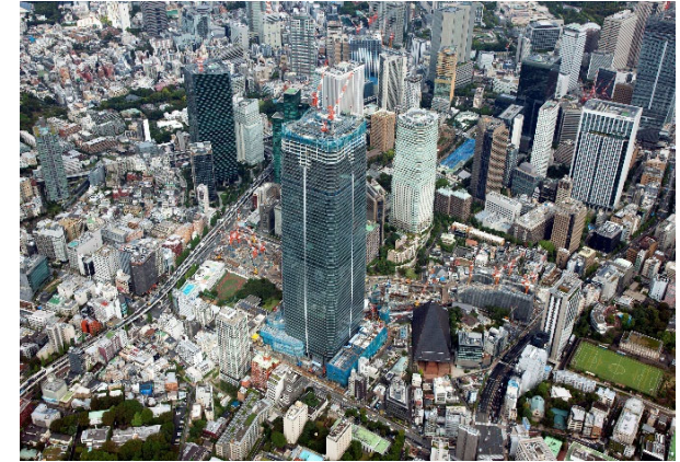
A District construction site (October 2022)
