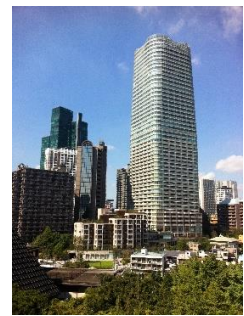
ARK Hills Sengokuyama Mori Tower (2012)
