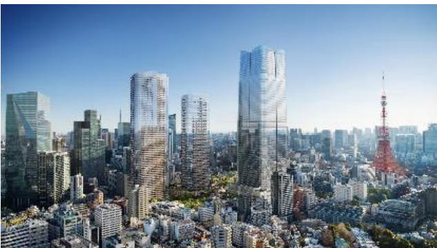
Credit: DBOX for Mori Building Co.
