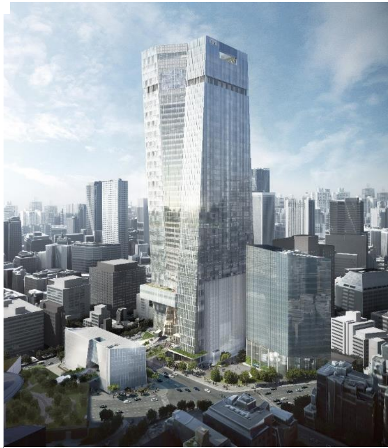
A-1 district: Toranomon Hills Station Tower
