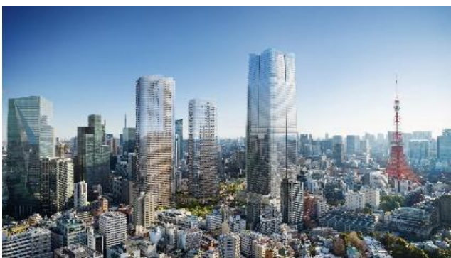
Credit: DBOX for Mori Building Co.
