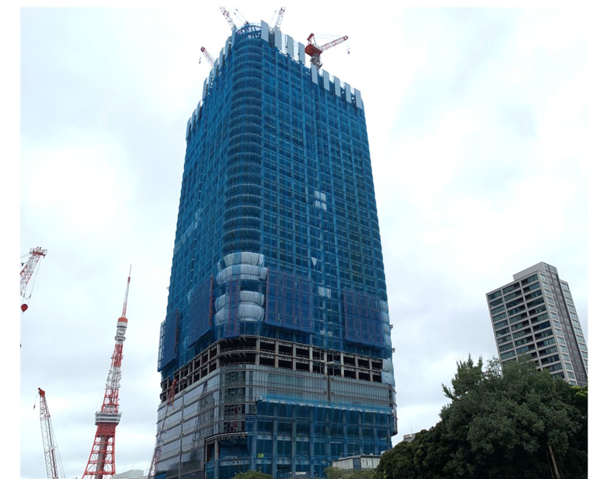
Construction site (A district; September 2021)
