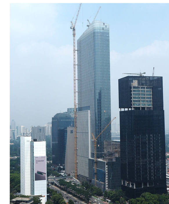
Construction site (September 2021)
