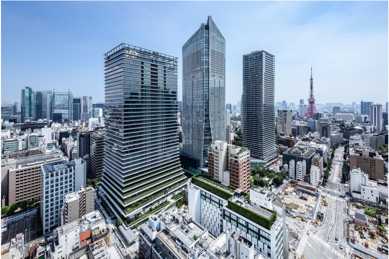
Current view of Toranomon Hills area (Photo taken in June 2020)
