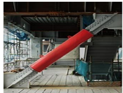
Buckling-restrained Brace
