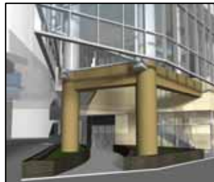
First floor pilotis
