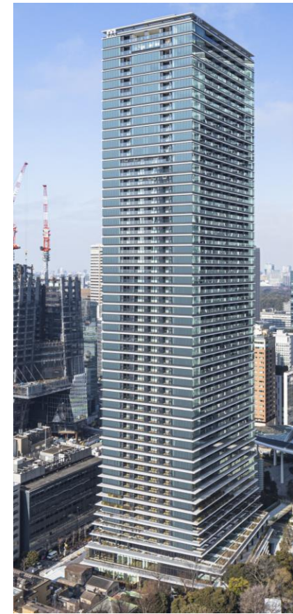
Toranomon Hills Residential Tower
