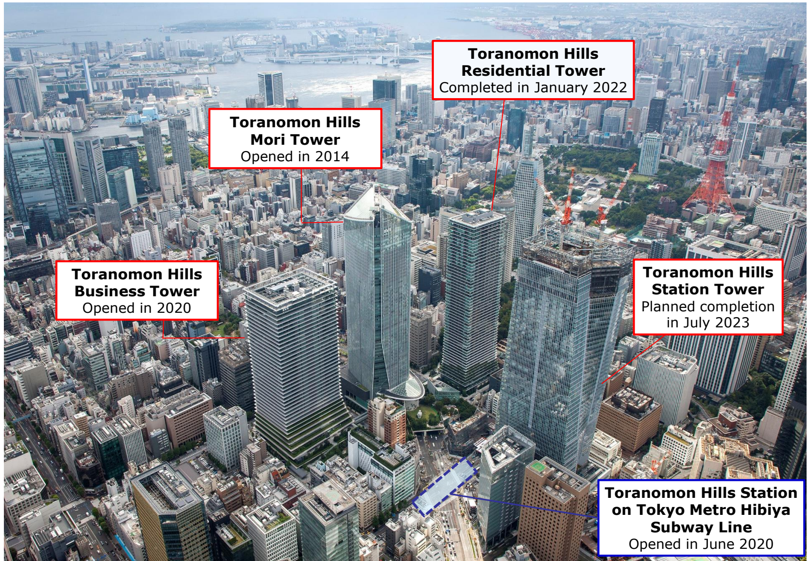
Construction site of Toranomon Hills Area Project (October 2022)
