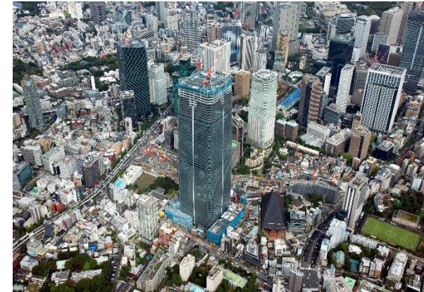
A District construction site (October 2022)
