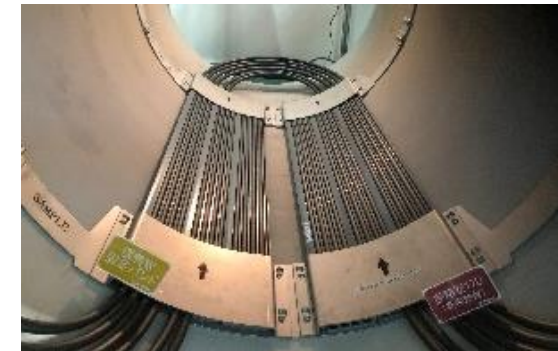
Heat exchanger in sewerage pipeline (image)
