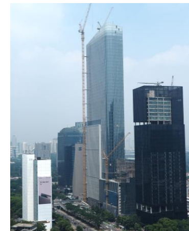
Construction site (September 2021)
