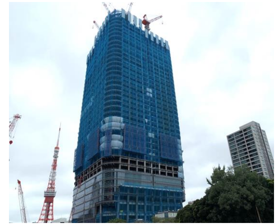
Construction site (A district; September 2021)
