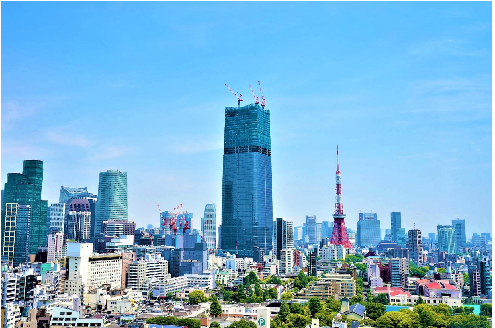
Construction site of Toranomon-Azabudai Project (May 2022)
