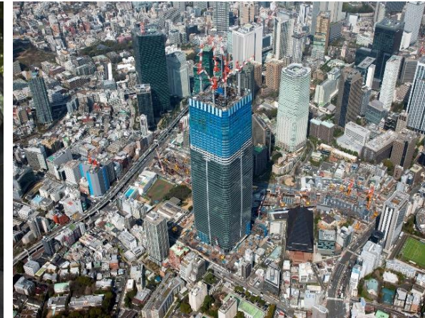
A District construction site (March 2022)
