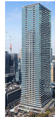
Toranomon Hills Residential Tower
