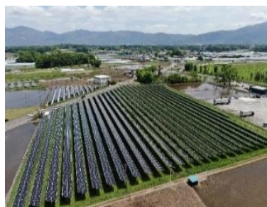
Mori Building Chikusei City Kuwayama Agricultural Solar Power Plant
