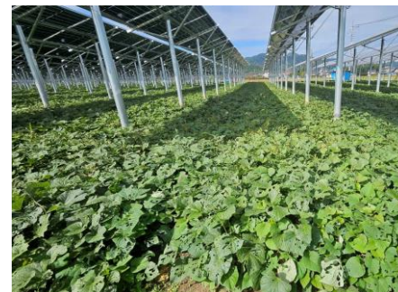
Mori Building Tochigi-shi Miyamachi Farm-scale Solar Power Plant
