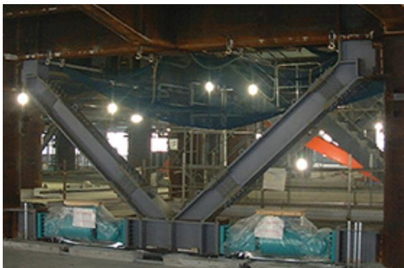
Semi-active oil dampers
