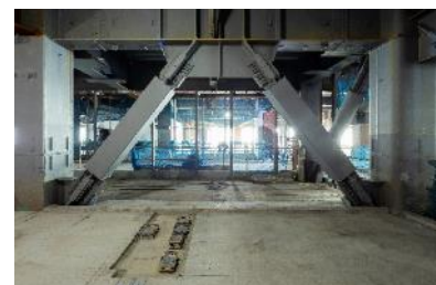
Buckling-restrained brace
