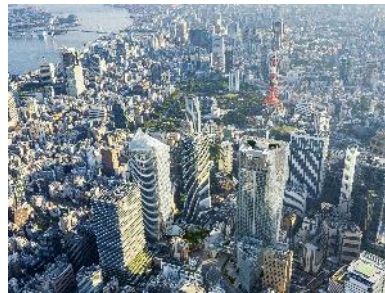
Toranomon Hills (completed October 6, 2023)
