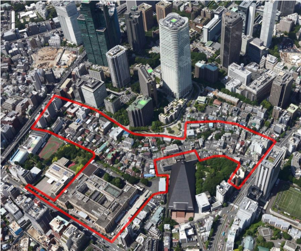
Aerial view of the project site before redevelopment
