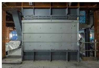
Viscous wall damper
