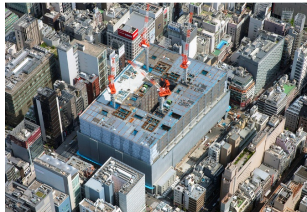
Photo of the site as of April 25, 2016
